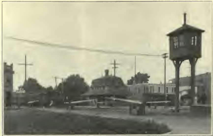
FIG. 255. GRADE CROSSINGS. Stony Island Avenue highway crossing of the South Chicago Branch of the Illinois Central Railroad.
